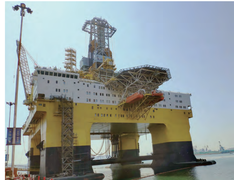
Figure 5 Construction Drilling Platform Blue Whale II
